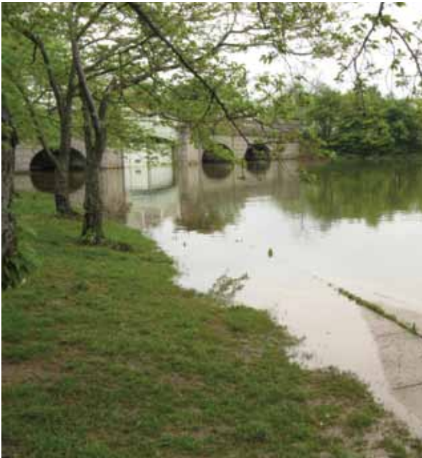
High water flooding in Washington, D.C.
