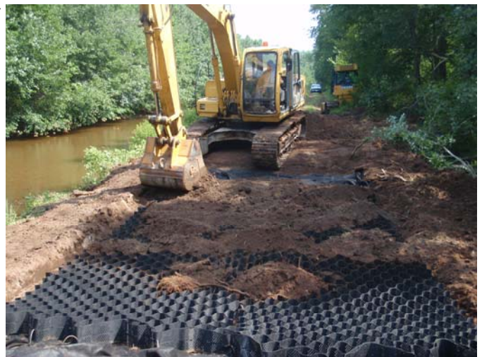
Restoring Tax Ditch Connection to Forested Wetland Floodplain (WMAP)
