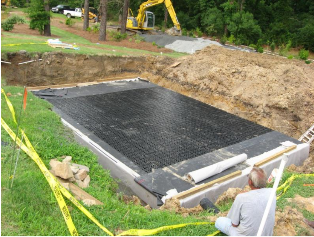
Figure 2-5. Below-ground cistern.
