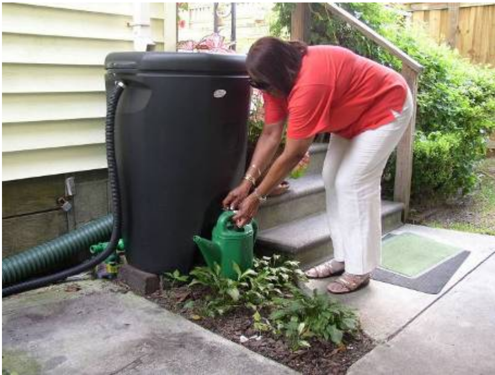
Figure 2-6. Residential rain barrel.
