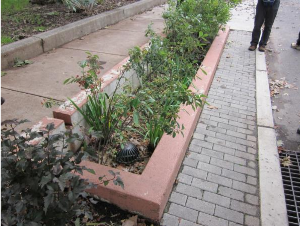
Figure 2-9. Roadside flow-through planter.
