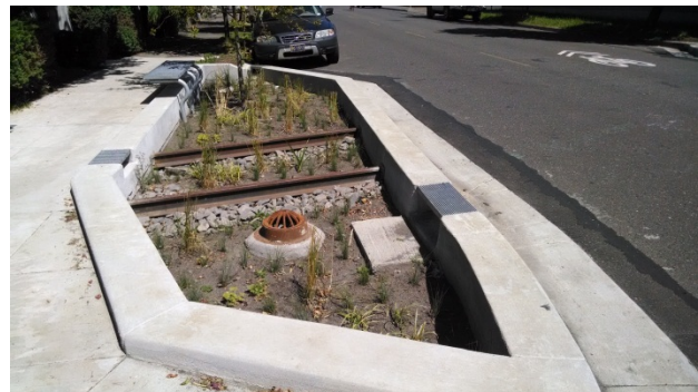
Figure 2-8. Bioretention planter box.
