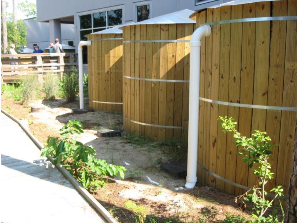
Figure 2-3. Wood wrapped cisterns.
