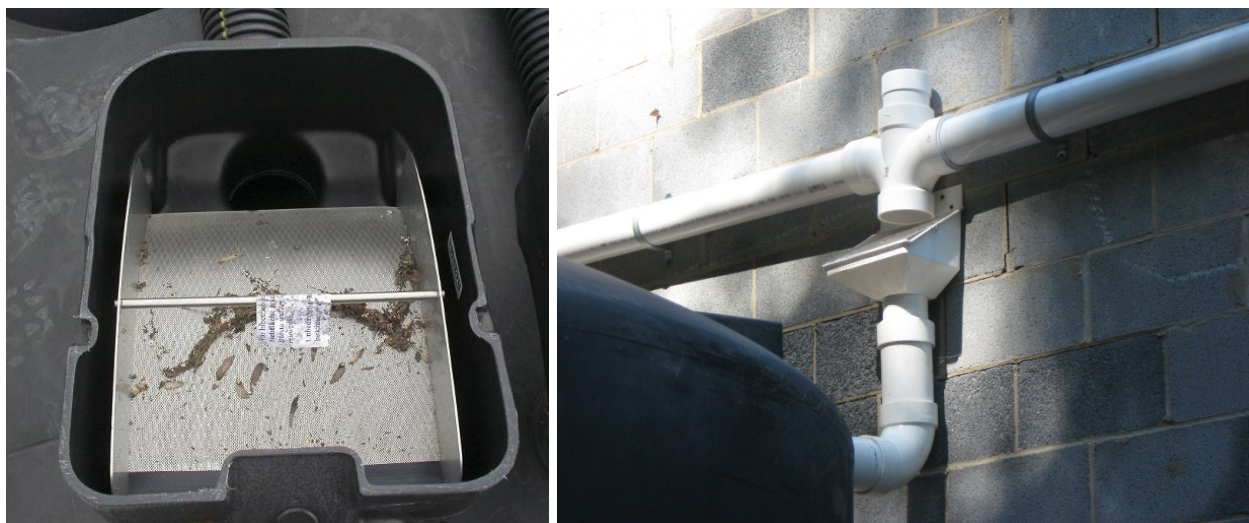
Figure 3-9. Self-cleaning inlet filters.
