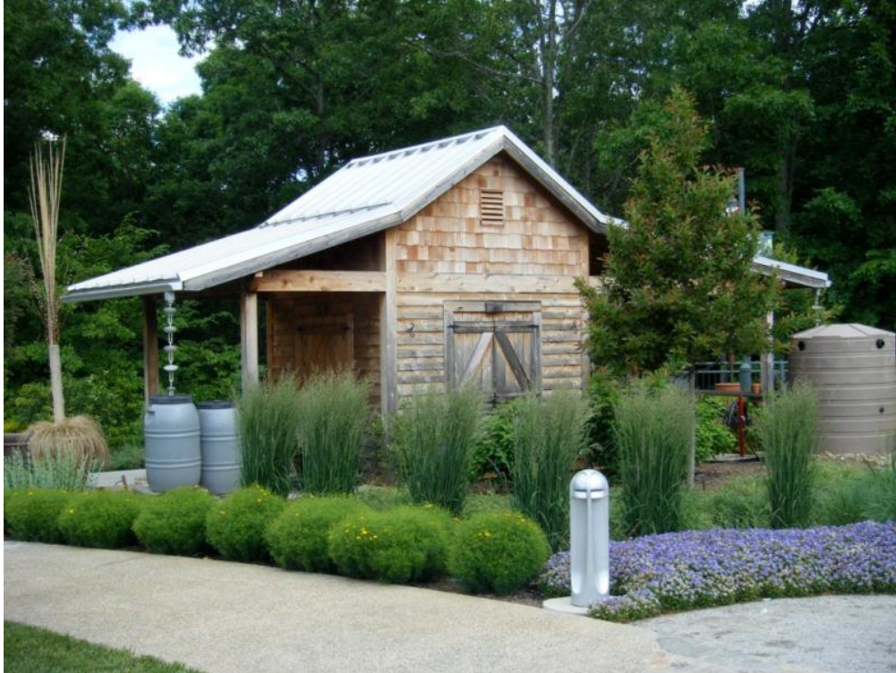
Figure 2-7. Rain barrels adequately sized for contributing roof area.
