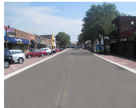
Permeable Pavement in parking area Source: Suzy Cho, LID Center
