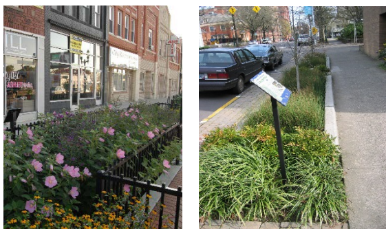
Lansing, MI roadside bioretention. Source: Robert Domm, Tetra Tech
