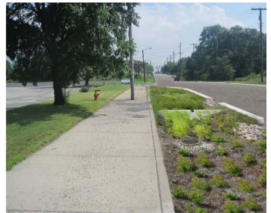
Bioretention along road Source: Suzy Cho, LID Center
