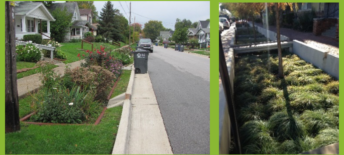
Cities like Toledo, OH (left) and Houston, TX (right) use green infrastructure along local streets to soak up stormwater. Sources: Dan Christian, Tetra Tech (left); Anne Thomas, Tetra Tech (right)
