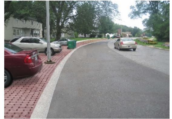
Permeable Pavement in parking area Source: Suzy Cho, LID Center
