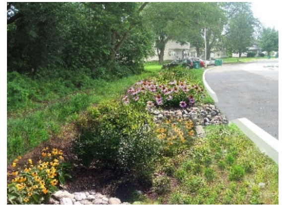
Bioretention along road Source: Suzy Cho, LID Center
