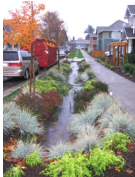
Roadside bioretention. Photo: MIG|SVR
