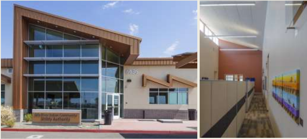
Gila River Indian Community Utility Authority building and interior. Photos: David Eisenberg
