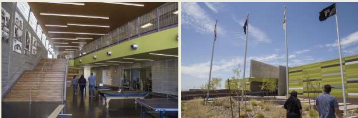
GRIC Hashan Kehk District 2 Service Center/Multipurpose Building. Photos: David Eisenberg
