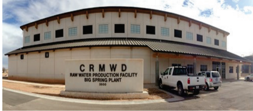
Figure A.5-1. CRMWD raw water production facility (Source: TWDB, 2015)
