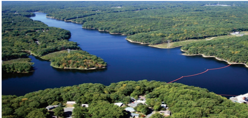
Figure A.7-1. Aerial view of the Occoquan Reservoir (Photo Credit: Roger Snyder, Manassas, Virginia)
