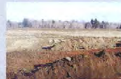
Circle drive restoration site at beginning of restoration construction.
