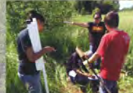
Installing monitoring wells.
