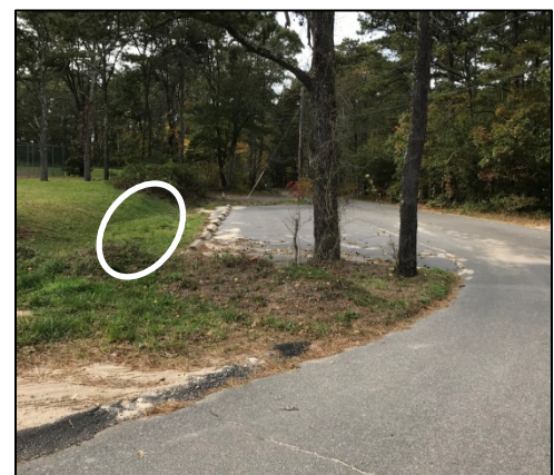
Infiltration BMP Behind Parking Area
