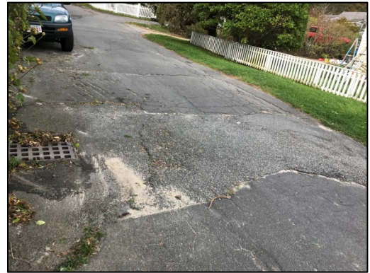
Catch Basin / Potential Swale Location
