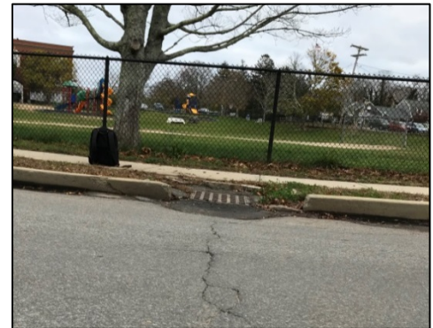
Catch Basin at School Curb
