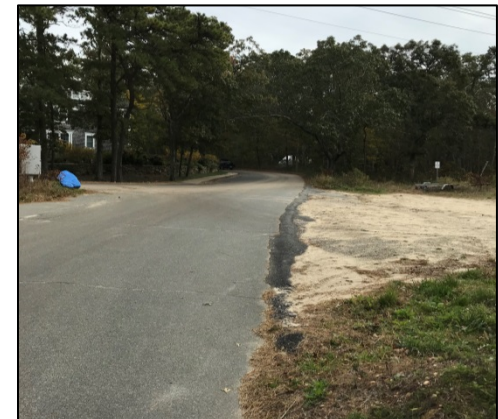
Lake Street Berm above Tennis Courts
