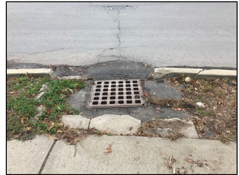
Catch Basin to Catch Basin
