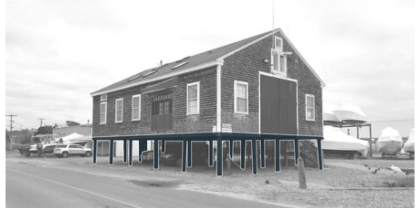
**Image:** *Shipyards at 100 Lagoon Pond Road.* Some properties in the Village of Vineyard Haven have begun to elevate service buildings in the waterfront.
