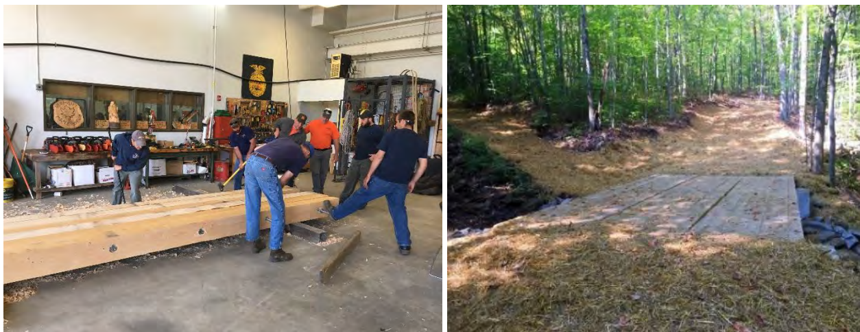
Figure 21. Left: Portable skidder bridge workshop; Right: Portable skidder bridge in Addison used at logging operation to avoid erosion at stream crossings (Source: Department of Forests, Parks and Recreation)
