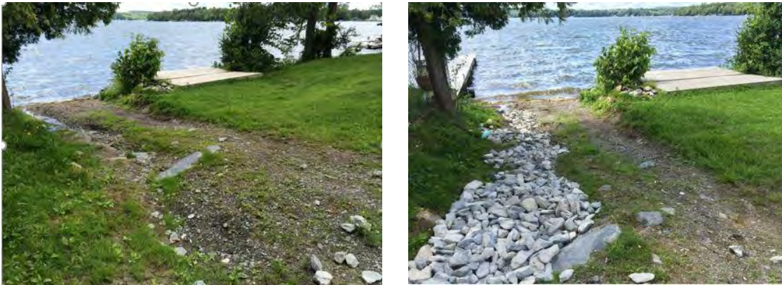
Figure 34. Before (left) and after (right) removal of the Mill Brook Dam in West Windsor, completed by Southern Windsor County Regional Planning Commission with funding from a DEC Clean Water Initiative Program grant
