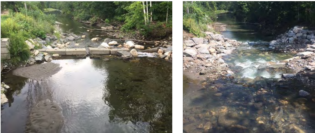
Figure 35. Before (left) and after (right) replacement of a deteriorating, 30-year old culvert with a bridge on Boulley Brook in Johnson completed by Vermont Department of Forests, Parks and Recreation with funding from a DEC Clean Water Initiative Program grant (clean water project sign posted during construction)
