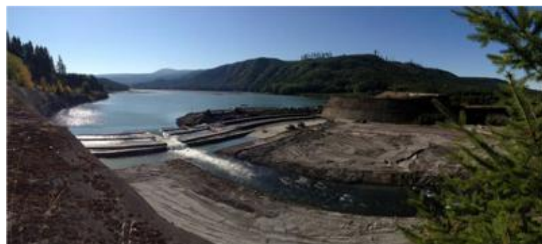
Photo 7-5 Sediment retaining structure on the north fork of the Toutle River, which eventually flows to the Cowlitz
