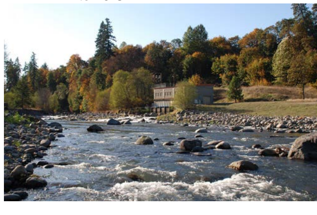
Photo 7-47 Hood River at the site of the former Powerdale Dam
