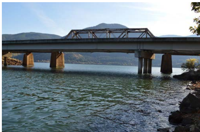
Photo 7-34 The confluence of the Little White Salmon River via Drano Lake flowing into the Columbia River
