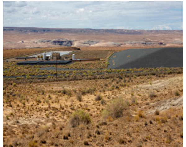
The Tuba City Disposal Site East of Tuba City, AZ.
