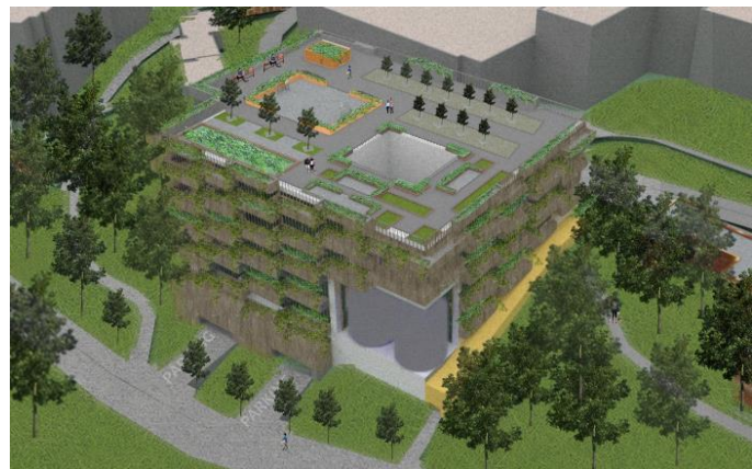
Figure 13: Site rendering of the proposed Upper Hillside Development. Most notably displaying the preserved basketball courts and recreational area on top of the garage's green roof. And exposed cisterns and terraced wall planters offer educational opportunities.
