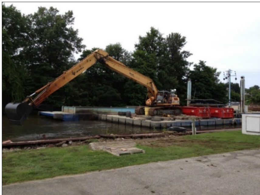
Figure 4: Dredging at Jack's Marine North Slip
