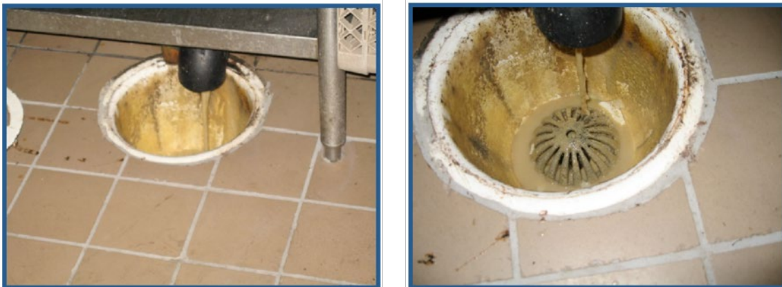
FIGURE 6. LIQUEFIED FOOD WASTE OUTPUT FROM A BIODIGESTER ENTERING THE SEWER SYSTEM
