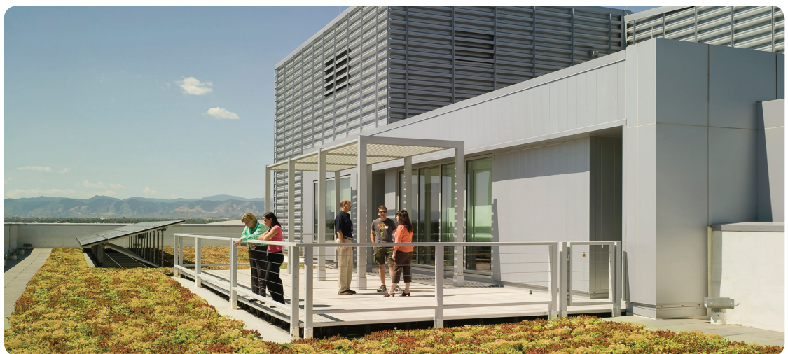
The green roof installed by EPA Region 8 provides welcome open space in the heart of the city. Photo courtesy of Greg Davis.
