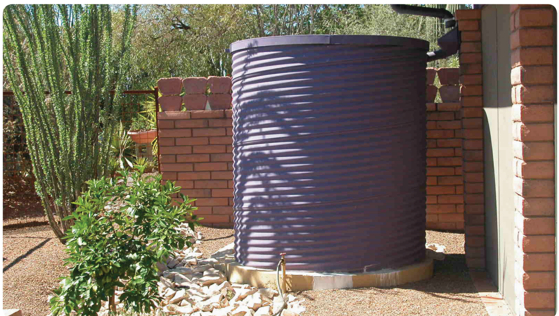
This rainwater cistern installed at a residence in Tucson, Arizona supplies water for citrus trees and a small vegetable garden, as well as native plants. Photo courtesy of Technicians for Sustainability.
