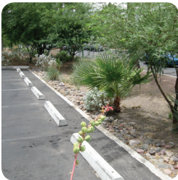
Passive rainwater harvesting in Tucson, AZ. Photo courtesy of Watershed Management Group.
