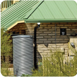
Active rainwater harvesting in Tucson, AZ.
