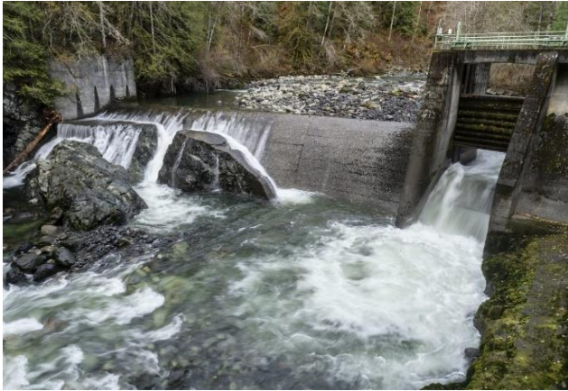
BEFORE DAM REMOVAL. PHOTOS: CITY OF BELLINGHAM
