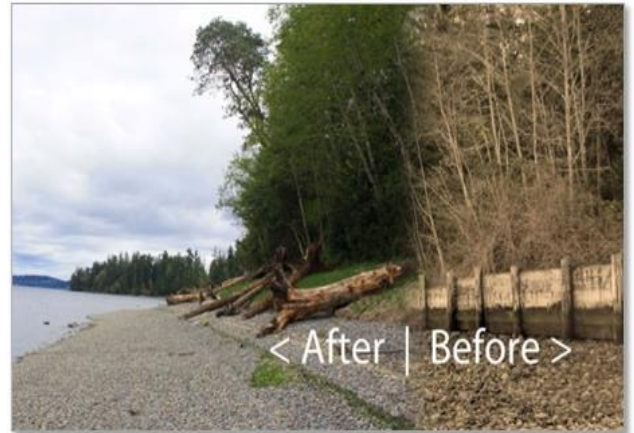
BEFORE AND AFTER BEACH RESTORATION USING A SOFT SHORE APPROACH. PHOTO: PUGET SOUND INSTITUTE
