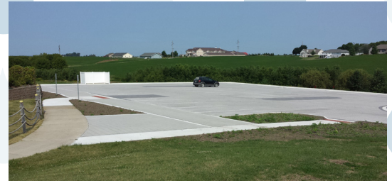
The Monona Aquatic Center parking lot after installation of permeable pavers.
