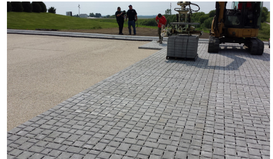
The contractor lays permeable pavers over layers of crushed stone.
