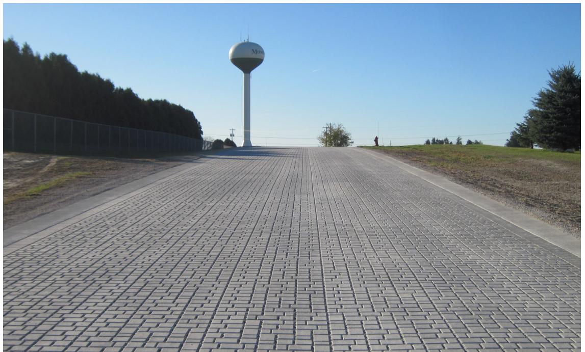
Permeable pavers were installed on a steep slope.
