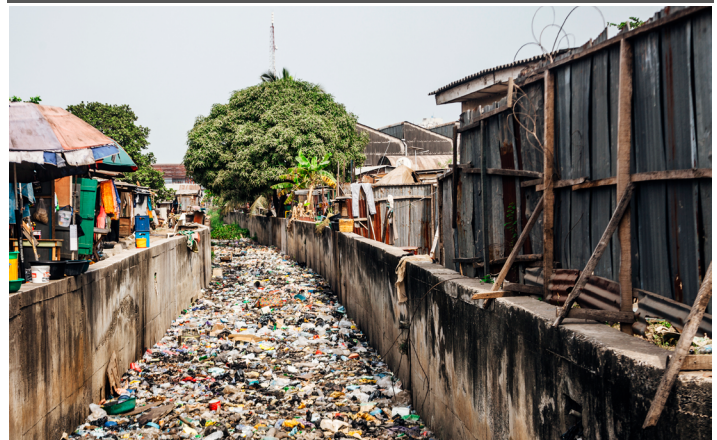
Exhibit 2. Waste in a community in Nigeria.
