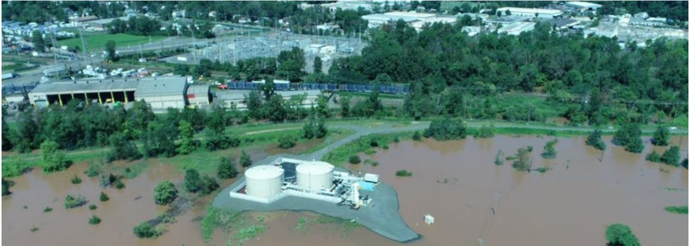
The groundwater treatment plant and storage tanks at the American Cyanamid Superfund site, constructed on elevated land outside the 500-year floodplain, avoided floodwaters in 2021. Photo Credit: Mark Schmidt.
