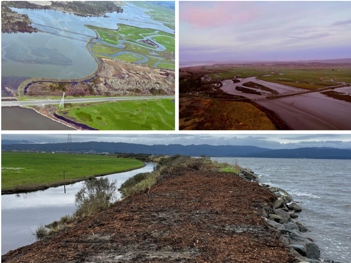
Figure 9: Views of Mad River Slough (northern Wigi-Humboldt Bay). Clockwise: Aerial view of the Slough and agricultural land during December 2023 King Tides in Wigi-Humboldt Bay. Aerial view of Mad River Slough at medium tide. View of the Slough (left) and Wigi-Humboldt Bay (right) from the top of an earthen dike. The dike is ~1ft away from overtopping and inundating the low-lying agricultural land that sits behind it.
