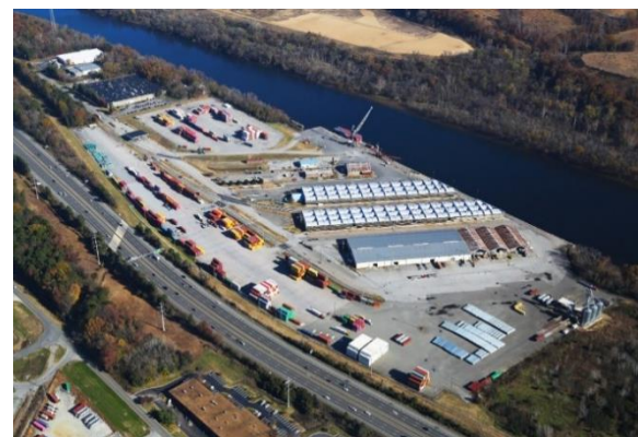
Figure 13. Richmond Marine Terminal
