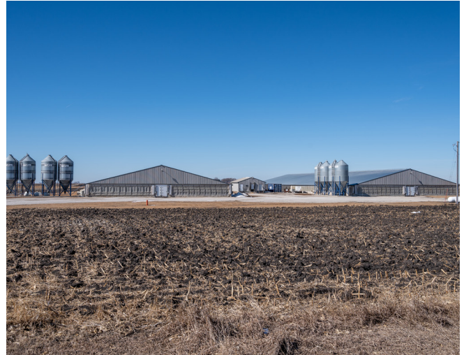
Two modern hog barns in Northwest Iowa.
