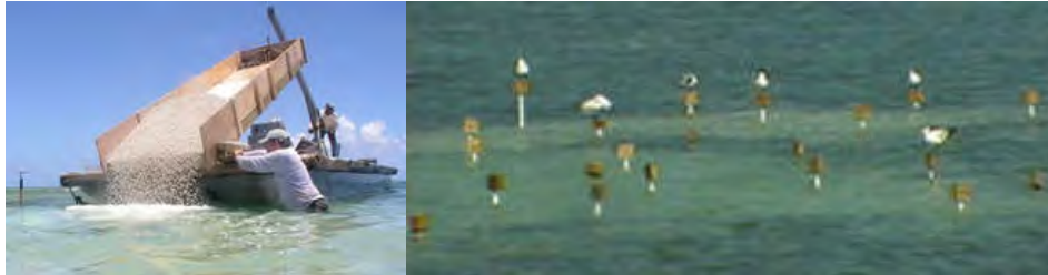
Figure 20. Seagrass restoration. The left image is the placement of sediment to return a blowhole to pre-injury elevation. The image on the right shows bird stakes placed in a restoration area (Both images are from www.darrp.noaa.gov ).
