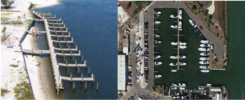
Figure 12. Sample Marina Images. The left image shows an example of an open water marina (provided by the Florida Marine Contractors Association), while the right image shows an example of marina contained within an upland cut basin (©2014 Google).
