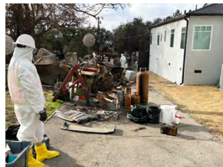
Empty canisters are marked and collected in front of cleared properties to be picked up at a later date
